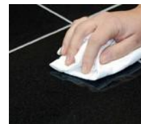
If necessary gently buff with a dry soft cloth or buffing machine.
