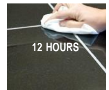
Buff away any excess moisture and allow the surface to dry. 12 HOURS
