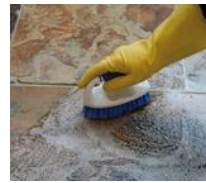
Agitate with a stiff brush or emulsifying pad to release the residual grout.
